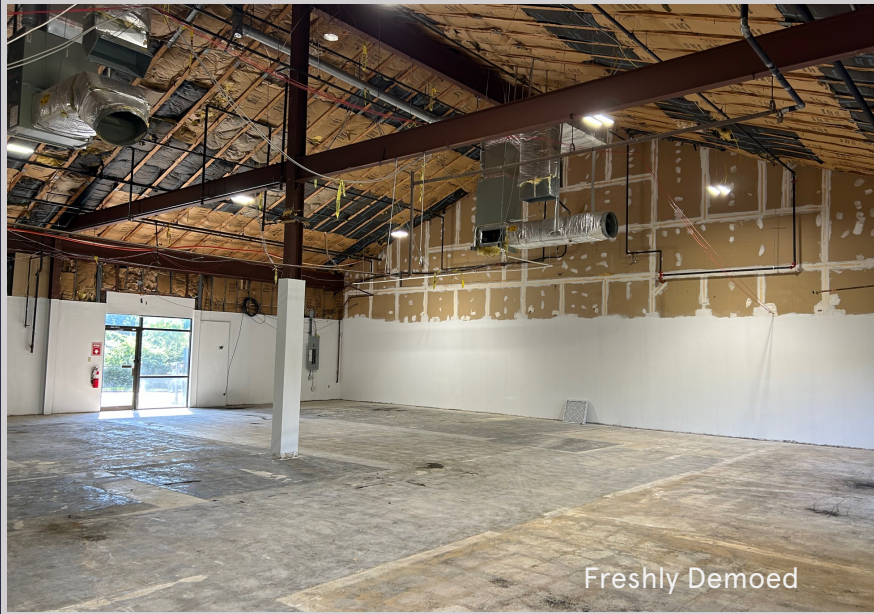
Loading Dock Interior
