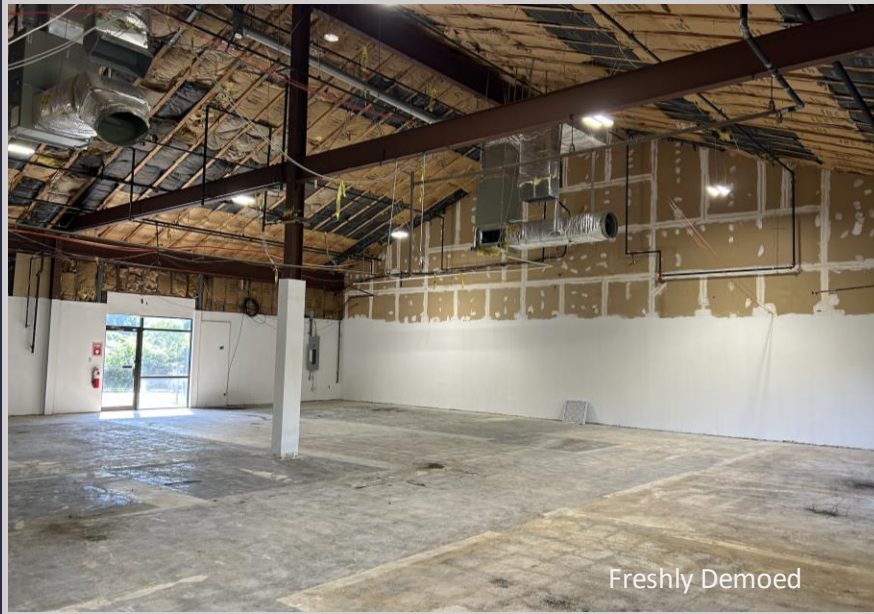
Loading Dock Interior
